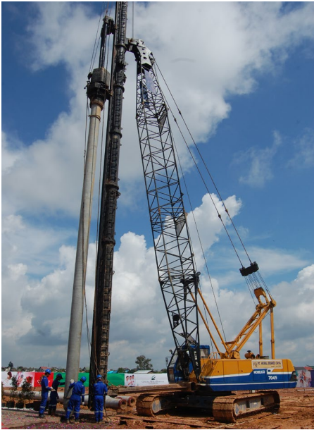
Suasana Ground Breaking CitraDream Hotel Yogyakarta
