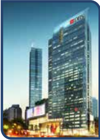
DBS Bank Tower – Jakarta Gold Rating Green Building Certification from Green Building Council Indonesia (GBCI)
