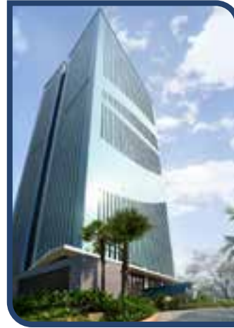
Citra Towers Kemayoran – Jakarta Final EDGE Certification from GBCI
